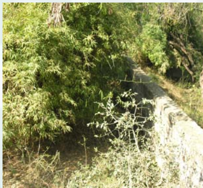
Stone check dam
